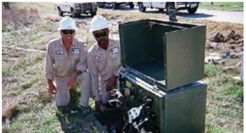
Rodney Wesley, right, started at TVEC doing right-of-way clearing on a brush crew, but soon made a career move into working on the power lines.
