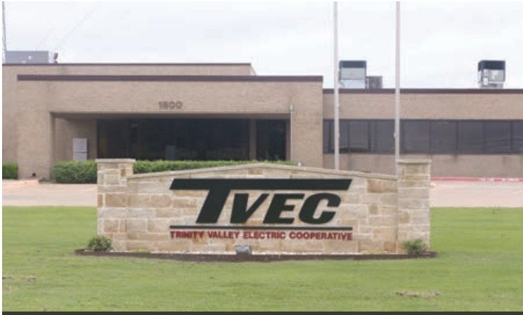
The current Trinity Valley Electric Cooperative headquarters building was built in the early 1980s.
