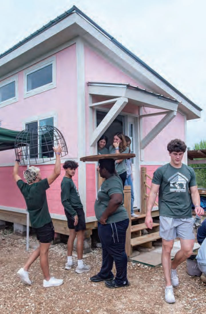
Kingwood Park High School students work on a tiny home.
