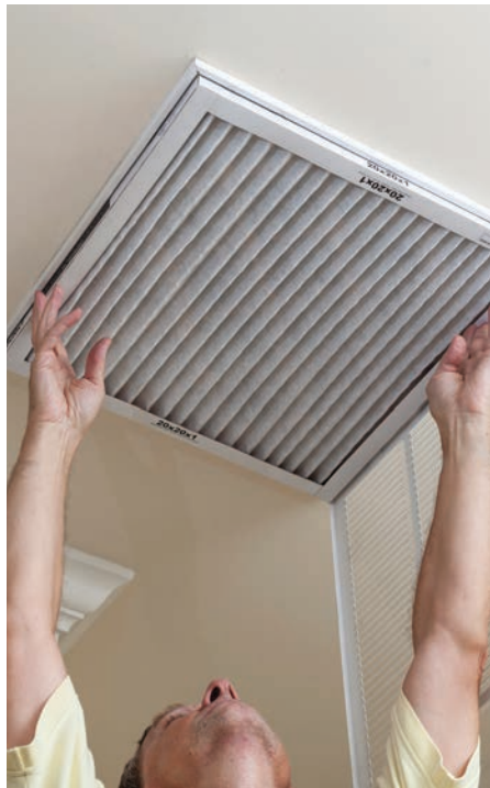
Your AC filter may be located in ceiling air returns, wall air returns in mobile homes, or in the attic air handler units.
