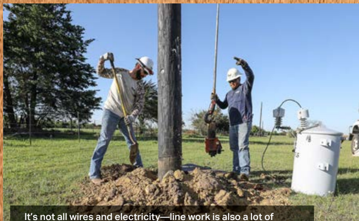
It's not all wires and electricity—line work is also a lot of heavy lifting and shoveling. Linemen Mitch Manthey and Hector Zarate work to relocate a pole while installing new service for a TVEC member.
