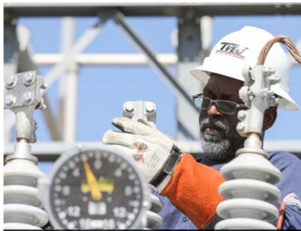
Lineman Jamie Davis works in the Mabank Substation as crews upgrade equipment June 5.
