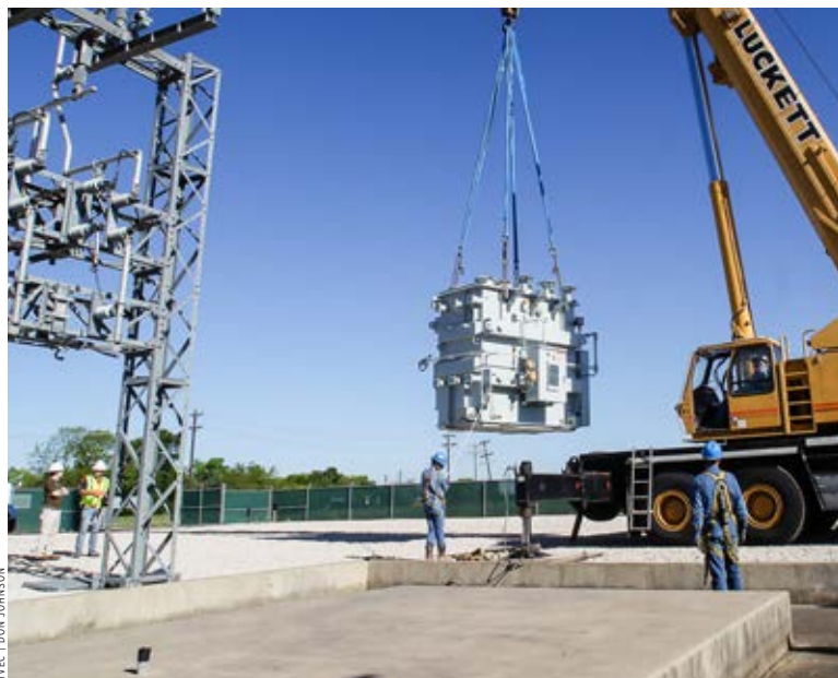
Workers hoist TVEC’s newest distribution transformer onto a waiting pad at the Marshall Substation north of Crandall. The unit will serve the rapid population and business growth in the Heartland, Forney and Crandall areas.
